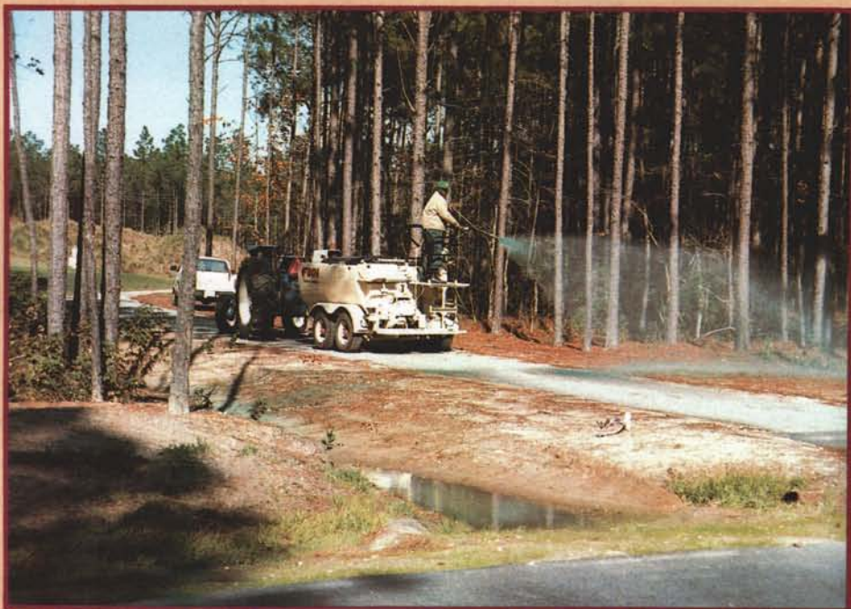
The plantation purchased a hydroseeder since seeding often had to be done between storms and a large amount of roadside seeding remained.
