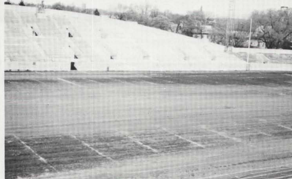
Worn-out football stadium field before renovation.
