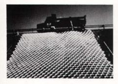
Enka Geomatrix Systems has acquired distribution rights to a soil stabilizer and erosion control material widely used in Europe. The product is a three-dimensional, semirigid geomatrix made of non-woven polyester fabric.
