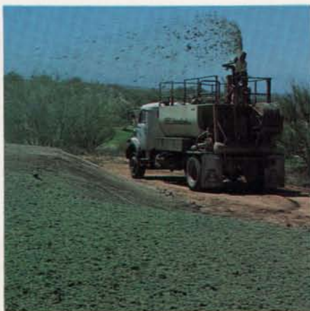
Over 70,000 sq. ft. of greens and tees were hydromulched in one day.
