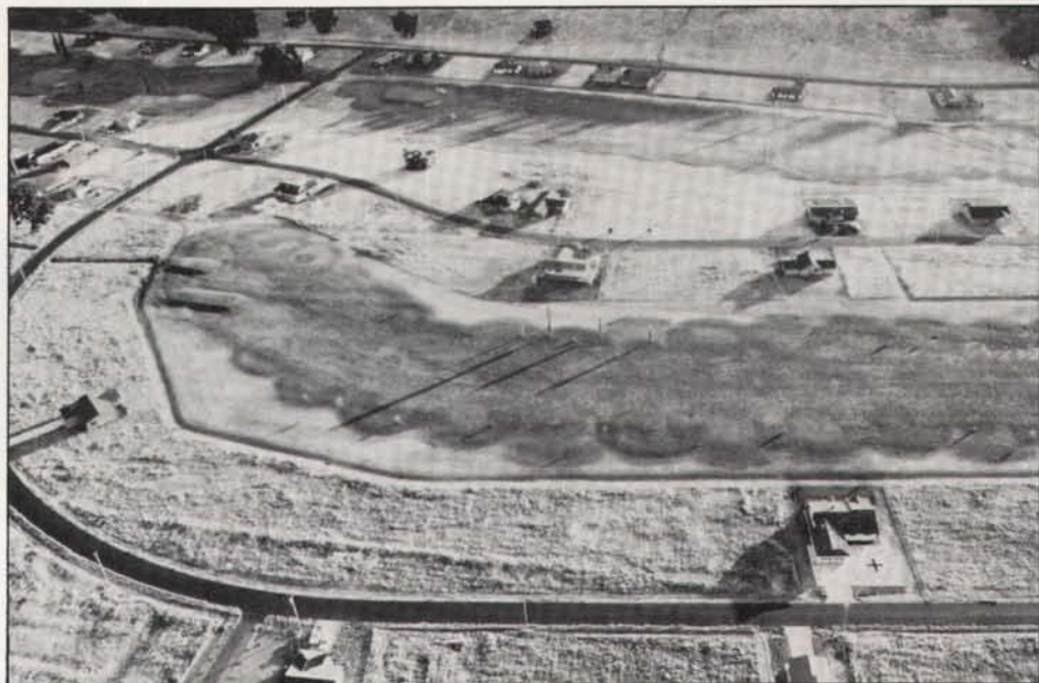
Improper irrigation design is evident on this new course, the center of a multi-million dollar real estate project. The obvious pattern in the turf will cause maintenance problems and golfer dissatisfaction.
