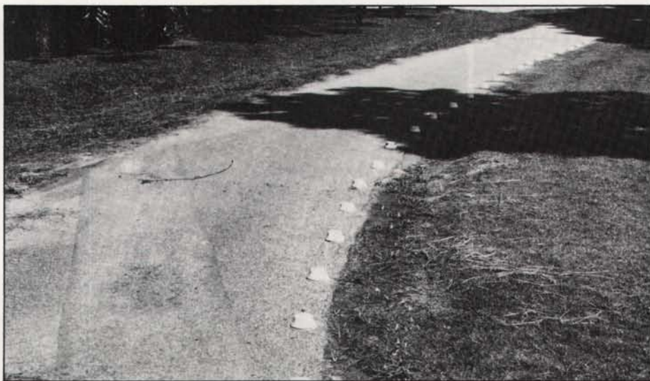
Traffic buttons on the edge of a cart path remind golf car drivers to stay on the path as they would stay in a highway lane.
