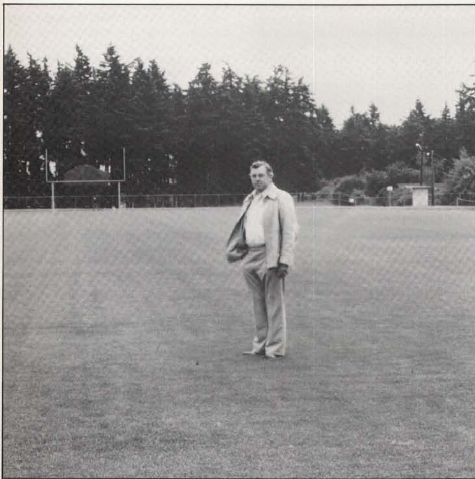
Dick Jenks stands on an Oregon high school field constructed with his Hi-Play sand rootzone, designed to handle the heavy winter rains of the Northwest.
