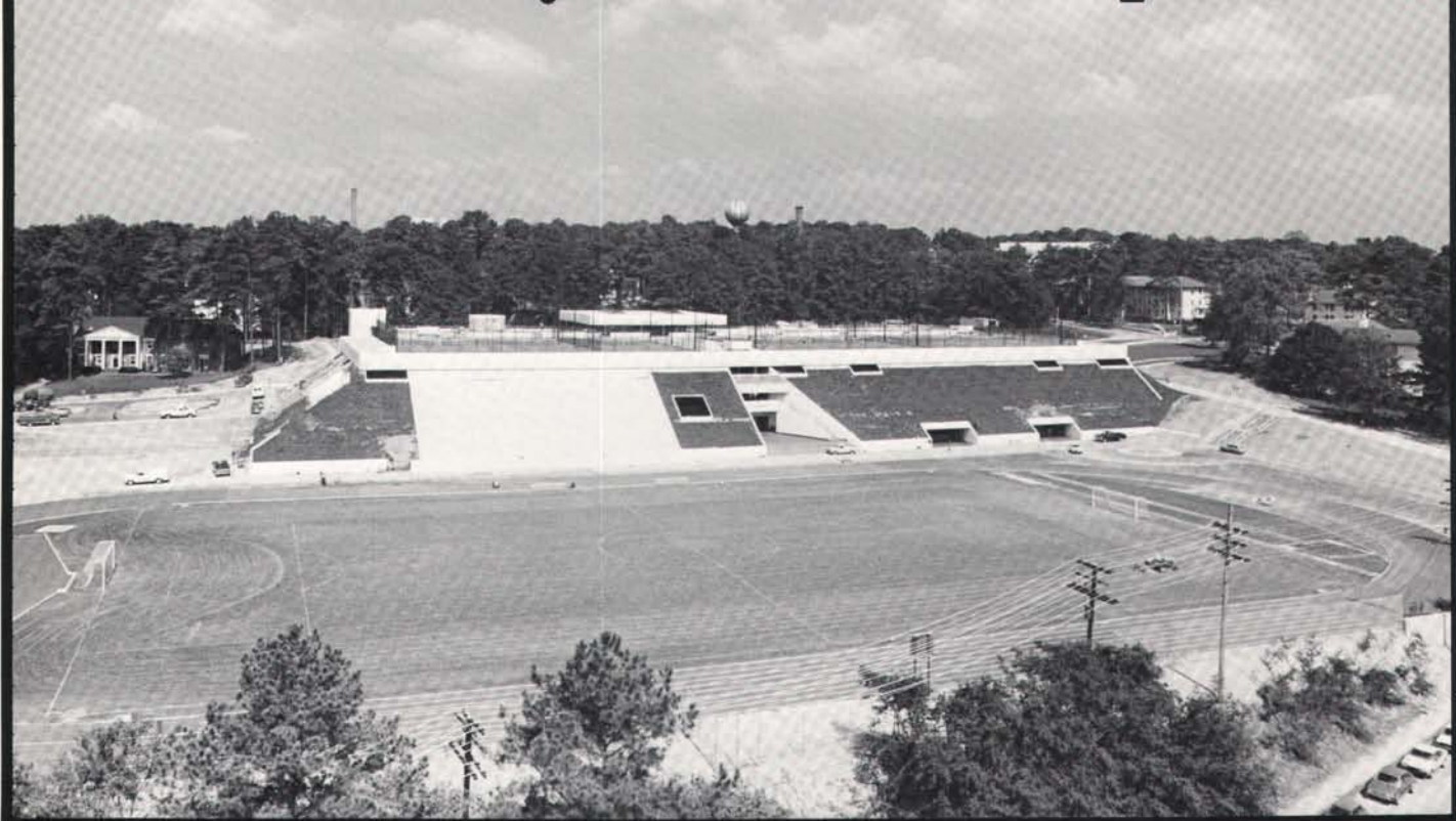
The George Woodruff Physical Education Center and soccer stadium was designed as a complete unit with the stands on one end of the building which is hidden by planted mounds.
